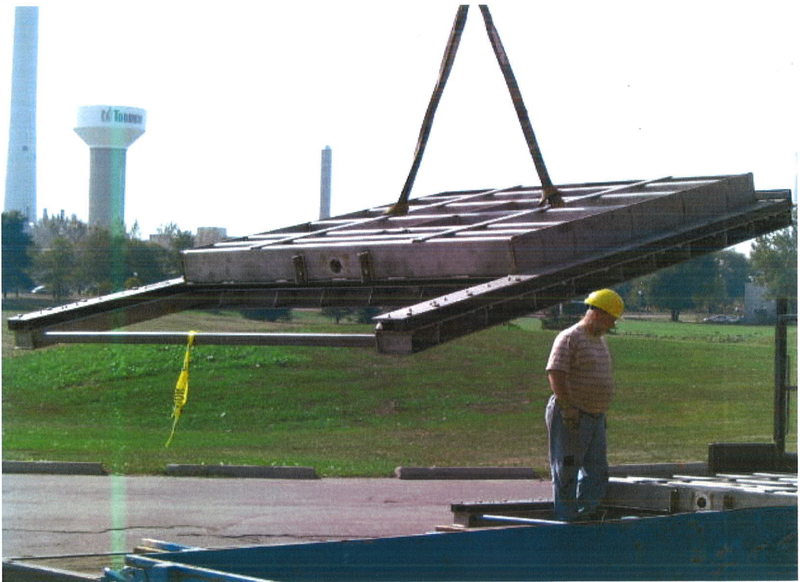
Dynamic Gate being supplied (Toronto)
