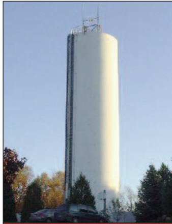
Mono Mills Standpipe
