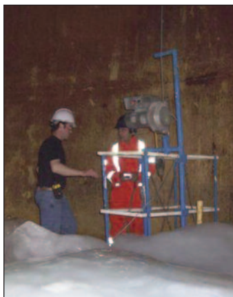
Contractors Working to Remove Ice From Tank
